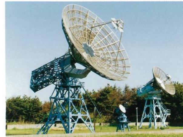
▲100/200 MHz(手前)と500 MHz(奥) 太陽電波観測用アンテナ Antennas for 100/200 MHz(front) and 500 MHz(back) Solar Observations
