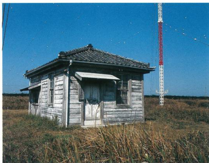
▲大正4年発足以来の1号庁舎、現在は平磯無線史料館 Building #1, constructed in 1915, is now being used as the Hiraiso Radio Historical Material Museum.
