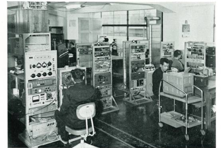
Test Room belonging to Research Section of Communication System.
