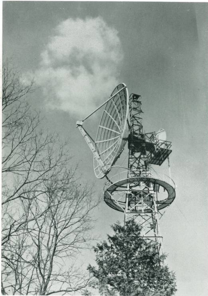
10 m Paraboloidal Antenna for Transmission on 600 Mc and 2120 Mc at Kokubunji Station, Tokyo.
