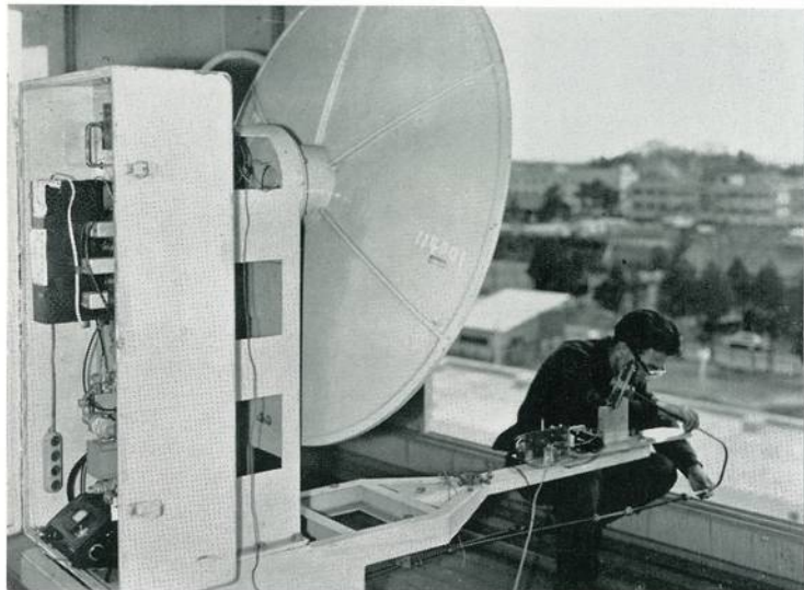
Off-set Paraboloidal Antenna for Transmitting 35 Gc Waves at Koku-bunji over 8.5 km Distance to the Tama-Hill.
