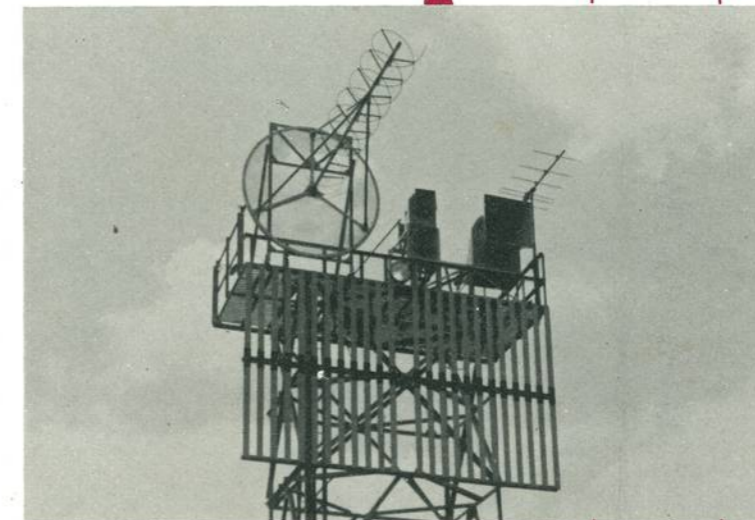
Collimation tower (8.8 km to the south-east from the main antenna).
