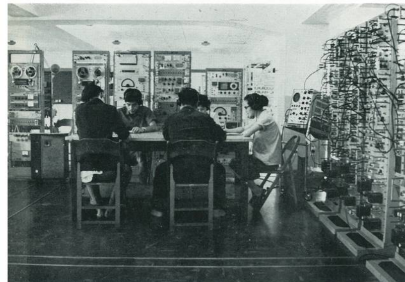
Testing Equipment for Communication Circuits, and Calibration Test for Measuring Apparatus
