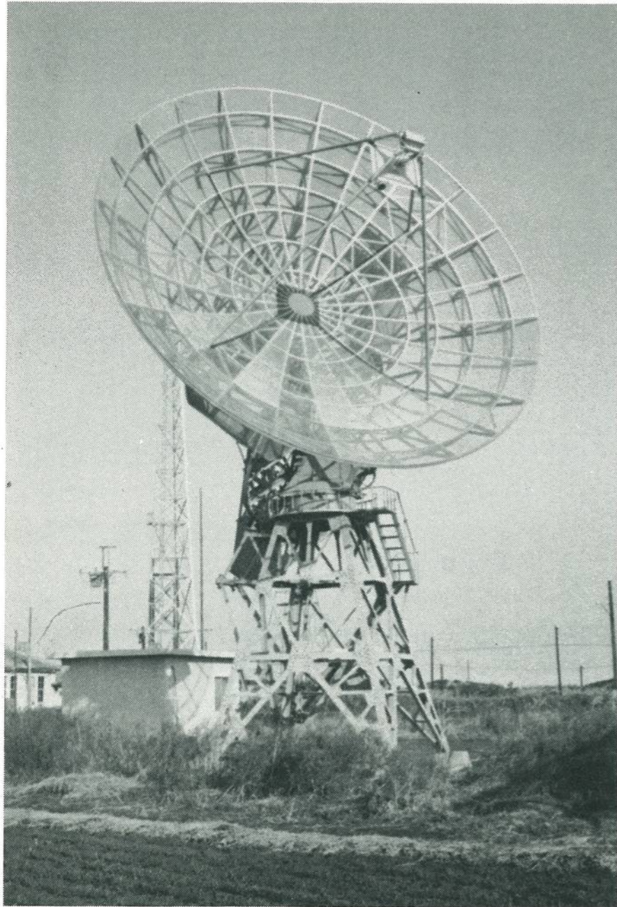
10 m parabolic antenna for 100 and 200 MHz
