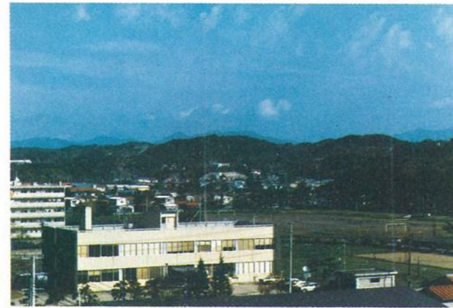
▲ AKITA RADIO WAVE OBSERVATORY 39° 43.5'N 140° 08.2'E 6-1, Tegata-Sumiyoshi-cho, Akita-shi, AKITA 010 JAPAN TEL. 0188-32-3767
