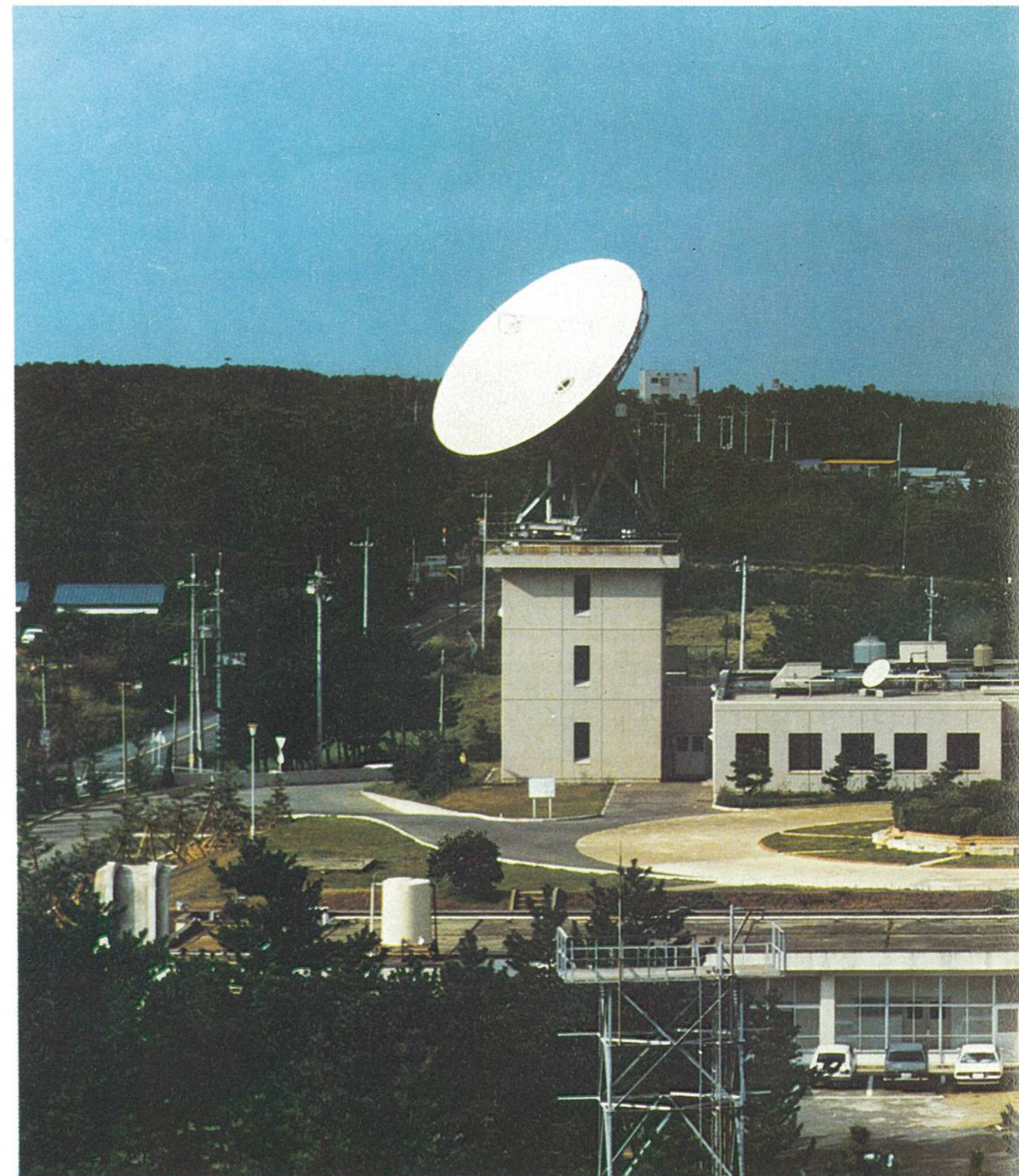
Main Transmit and Receive Station for BSE (left)
